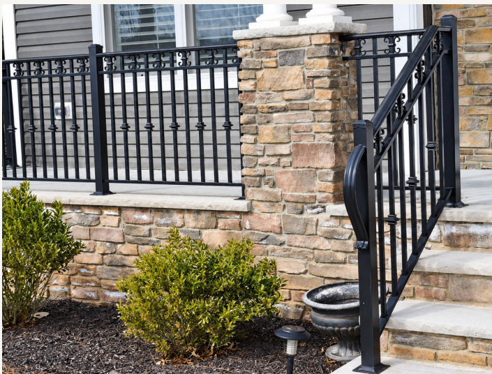
A-3 Top Molding with 2 1/2 in. posts, 3/4 in. pickets, collars every other picket, C-scrolls in top valance, and custom extra-large lambs tongue. Black.
