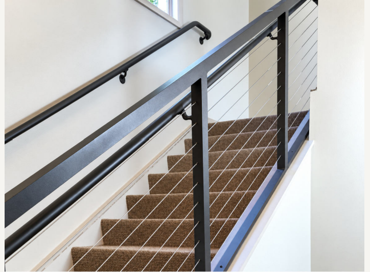
2 x 2 Aluminum Square Frame with 1/8 in. stainless steel cables, and graspable handrail. Textured Bronze.
