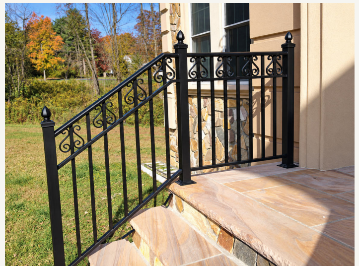
A-3 Top Molding with 2 1/2 in. posts, 3/4 in. pickets, S-scrolls in top valance, and acorn caps. Textured Black.
