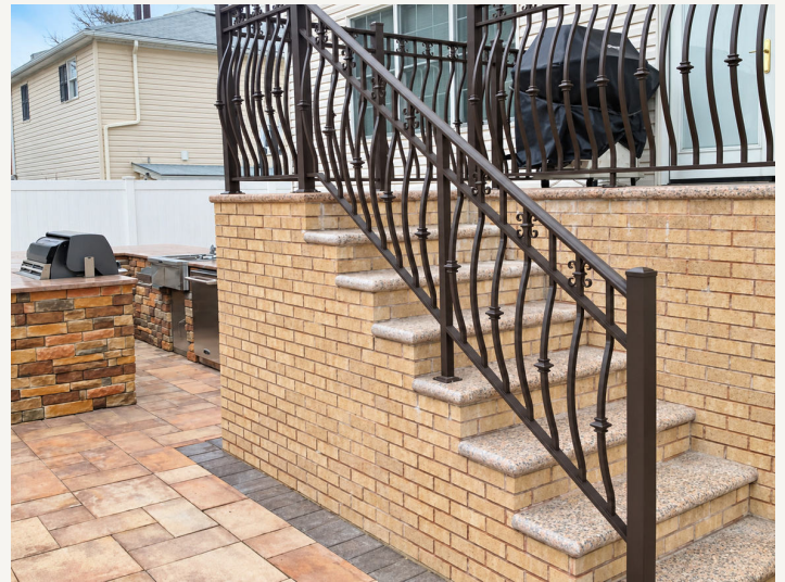
A-3 Top Molding with 2 1/2 in. posts, 3/4 in. bow pickets, and C-scrolls in top valance. Textured Bronze.
