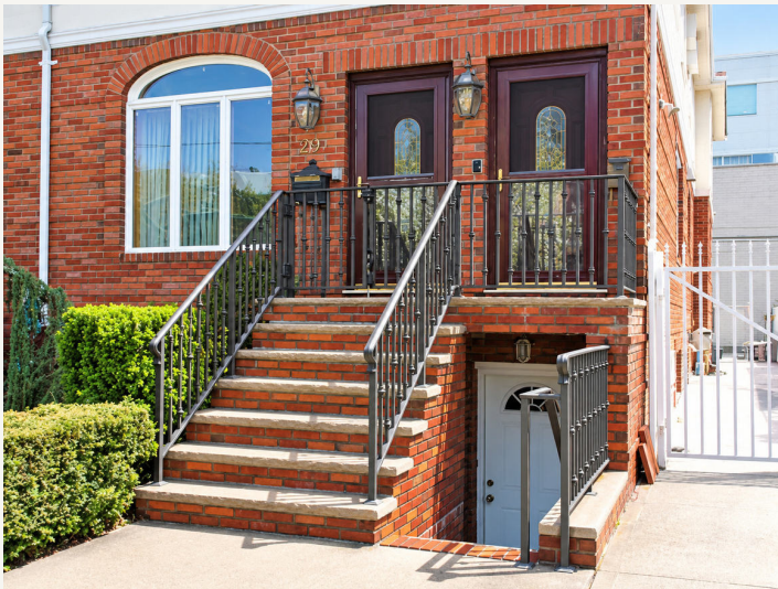
7500 Top Molding with 1 1/2 in. posts, 3/4 in. pickets, double single collars, and lambs tongue. Textured Bronze.
