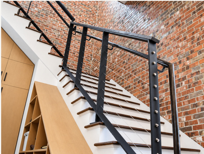
3 x 1/2 in. Cold Rolled Steel flat bar frame with 1/8 in. stainless steel cable, and custom wood top. Black.
